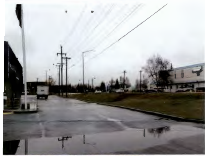
Oct 2019 Big Dipper Parking lot Drainage problem
