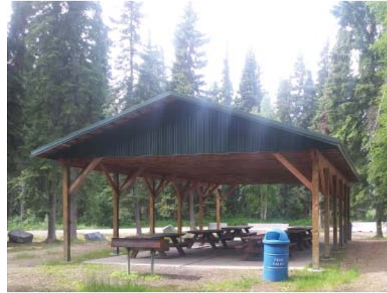
Shelter near the Noyes Slough Access - to be made ADA accessible
