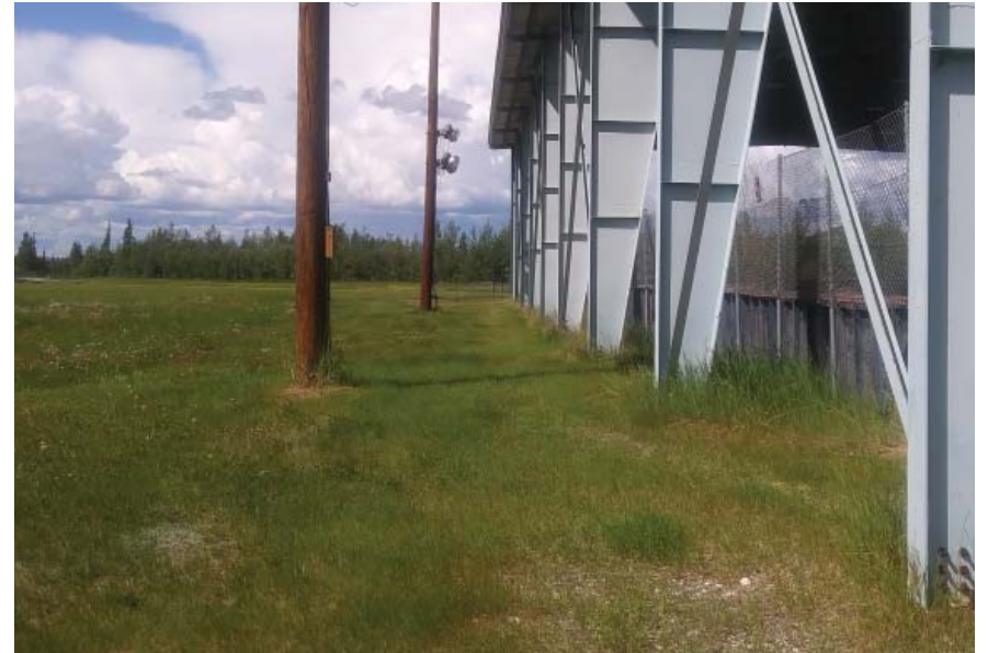
Existing lights outside of the structure.
