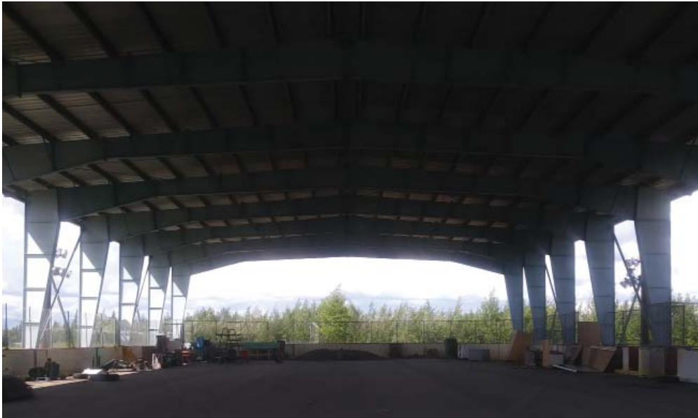
Metal Roof/Structure is in excellent condition.
